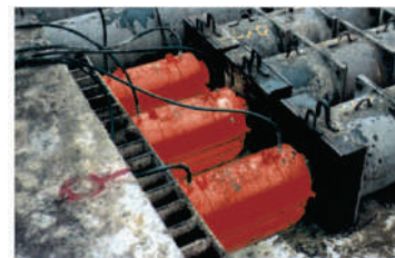
Three CLRG hydraulic cylinders are placed in parallel to push a prefabricated underground passage into place in segments
